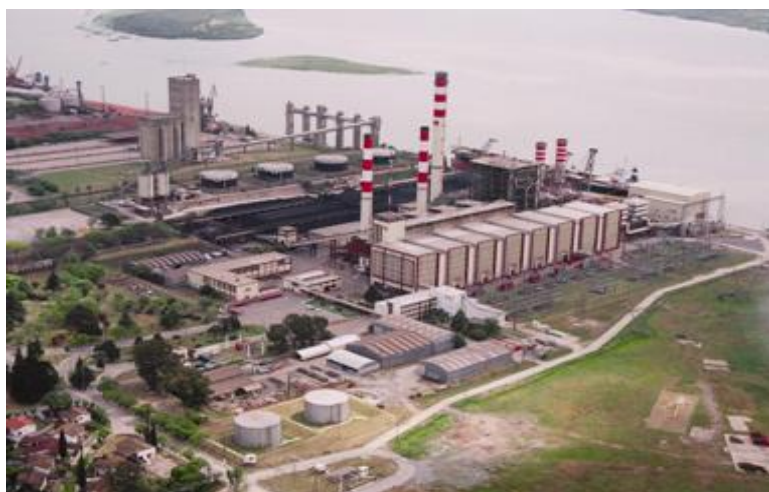
Central Termica Power Station
